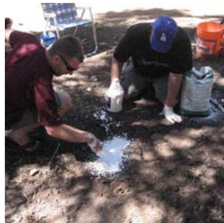
Cliff and Tom apply the splash coat of plaster.
